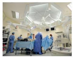
An octagonal unidirectional filtering ceiling with crystal curtains in one of the most modern operating theaters in Poland at Carolina Medical Center, executed by SAR PW in 2011
