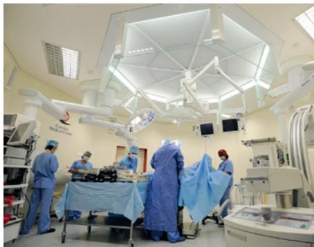
An octagonal unidirectional filtering ceiling with crystal curtains in one of the most modern operating theaters in Poland at Carolina Medical Center, executed by SAR PW in 2011
